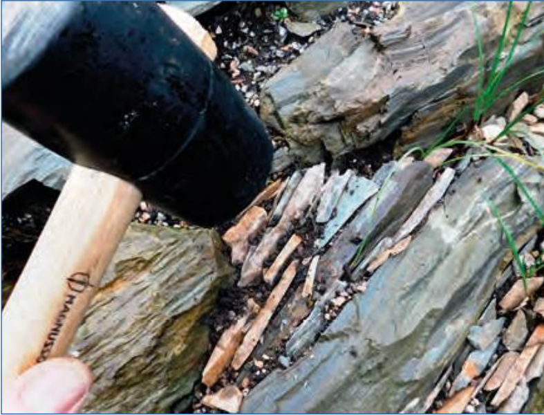
Rock sliver infilling with rubber mallet
